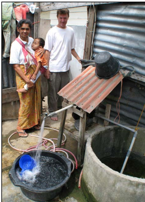
A WELL SPOILED BY THE TSUNAMI AND NOW USED ONLY FOR WASHING – VILLAGERS NEED TO EITHER BUY FILTERED WATER OR TRAVEL LONG DISTANCES TO FIND DRINKING WATER.
