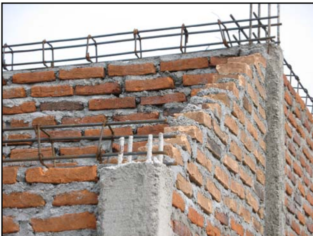
TYPICAL SITUATION OF INADEQUATE ANCHORING
