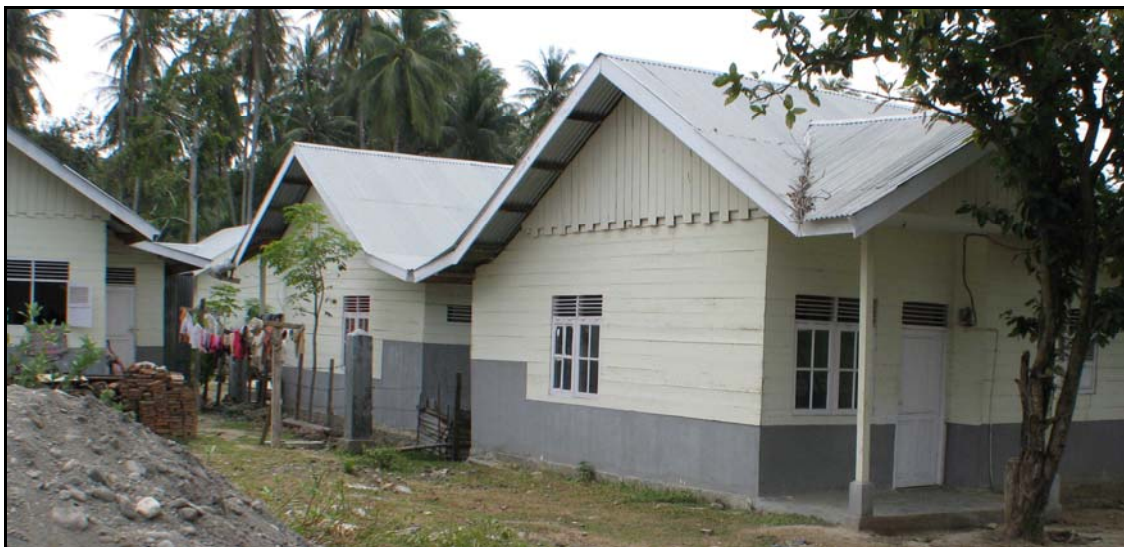
GOOD QUALITY BRICK AND TIMBER COMBINATION CONSTRUCTION, NOW CALLED SEMI-PERMANENT HOUSES
