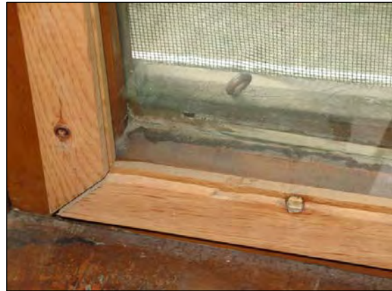
Knot in wood – wrong placement of screws. Open joint – knot and damage in profile.
