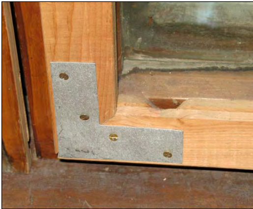
Knot in wood – wrong placement of screws. Open joint – knot and damage in profile.
