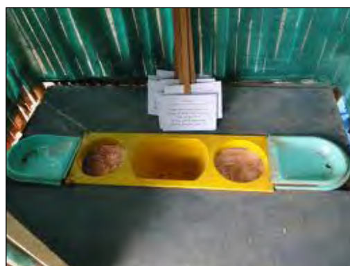
Left: Two complete UDDT units over two vaults below. The left vault below is closed for one year with a sheet of plywood on which the ash bucket is placed. Because the toilet is regularly washed, the plywood deteriorates and needs to be replaced periodically. A more durable water-resistant closing method is recommended.
