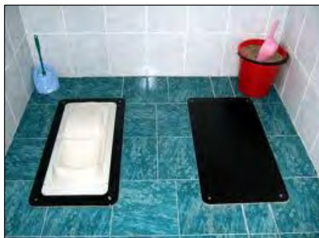
Left: A single squatting pan which is exchanged from one side to the other with the black cover when the vault is emptied. This saves some of the cost, especially if the plastic squatting unit is far more expensive than the cover.
