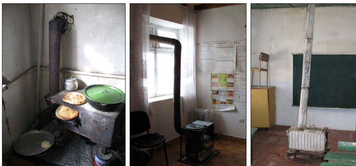
Three examples of chimneys going directly to the outside and removing all hot smoke gasses.
