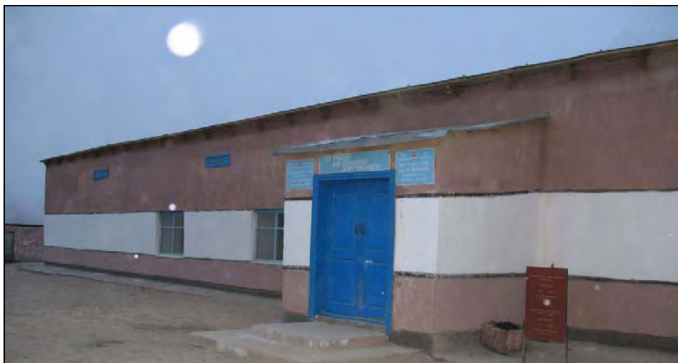
In this school the adobe cavity wall was constructed on the outside because of space requirements. Also the entire roof was insulated and a vestibule added to reduce the cold draft from outside.
